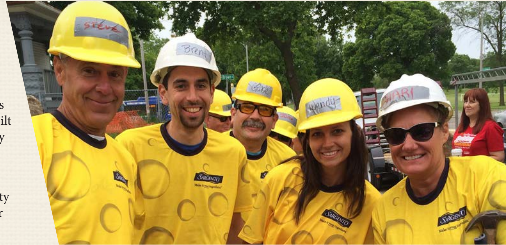
Lou Gentine stops by the Habitat for Humanity build site to lend a helping hand.
